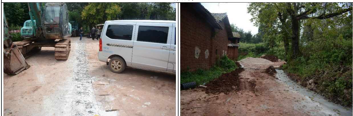
污水管管槽开挖
