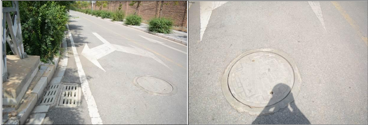
项目区周边雨水口及检修井
