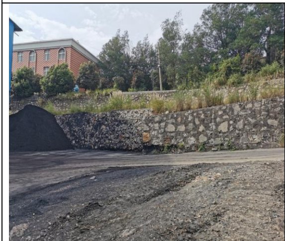
1#堆煤棚旁浆砌石挡墙现状
